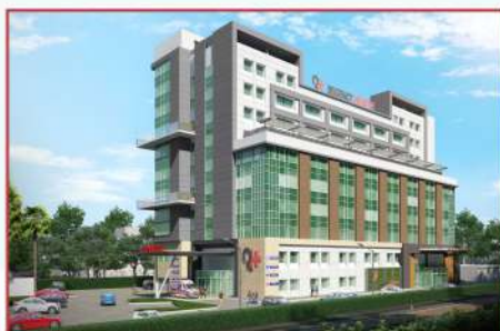
REGENCY HOSPITAL GORAKHPUR
